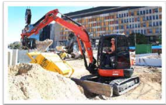
A construction worker backfills trenches as part of important stormwater infrastructure upgrades.
